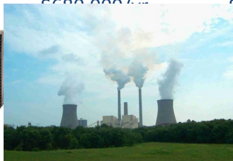
Conventional Power Plant 300 Megawatts
