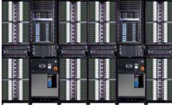
Open door view of 4 compute & redundant CDU racks
